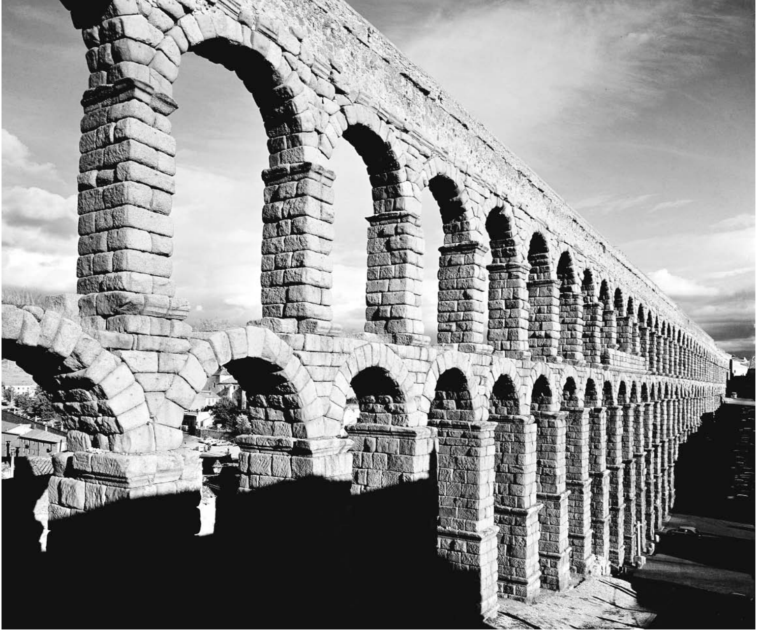
This granite aqueduct in Segovia, Spain, built without mortar or cement, has endured for 2,000 years, but pollution and age are slowly deteriorating it.
