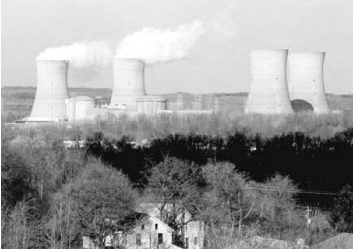
Two of the four cooling towers at the Three Mile Island nuclear plant stand idle, reminders of America's worst nuclear accident, which occurred in April 1979.
