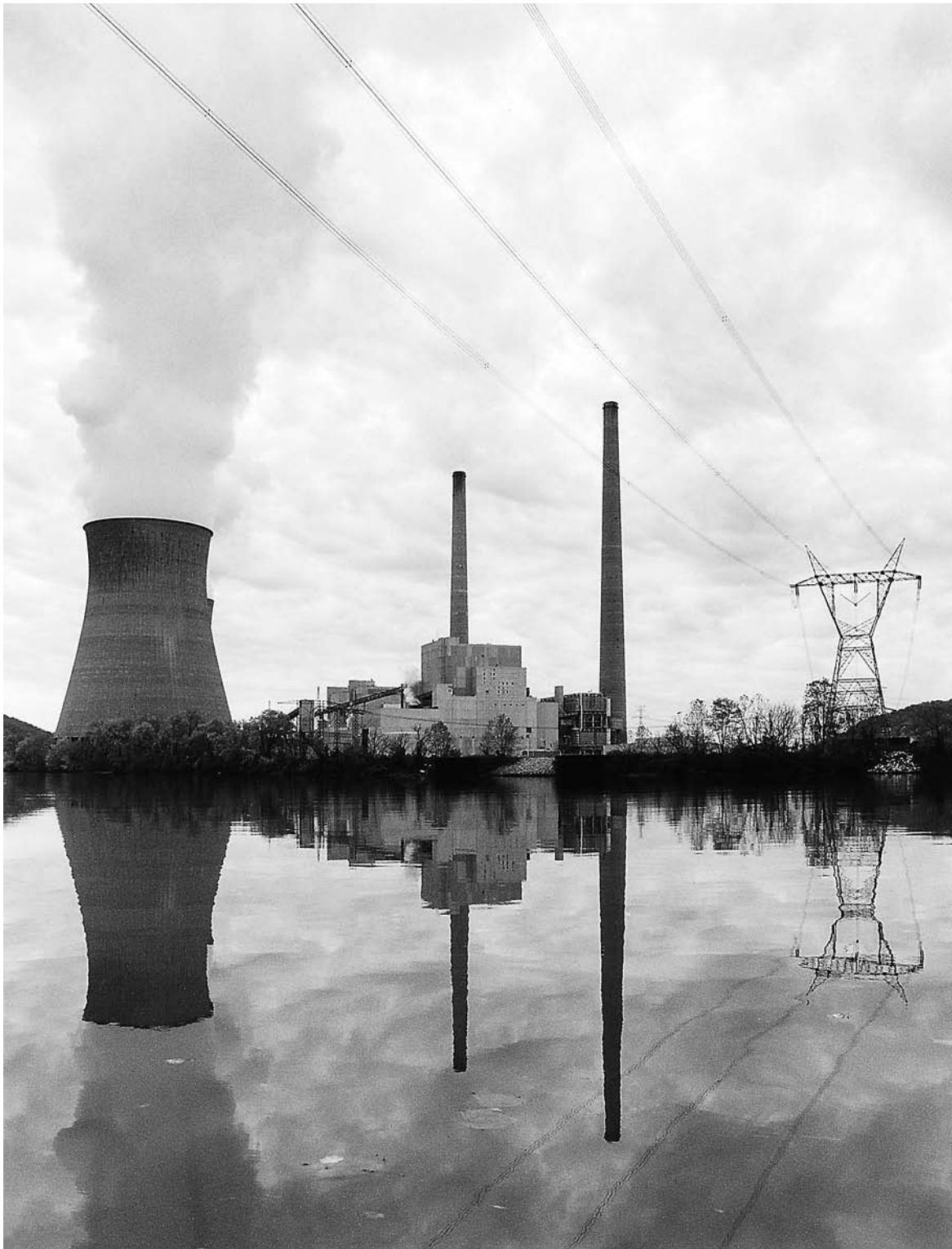
Interconnected power grids carry electricity across the United States from facilities such as this coal-fired West Virginia plant. In 2003, a plant failure in Ohio cascaded into a blackout that affected 50 million people. A key cause: Three overburdened power lines came into contact with untrimmed trees.
