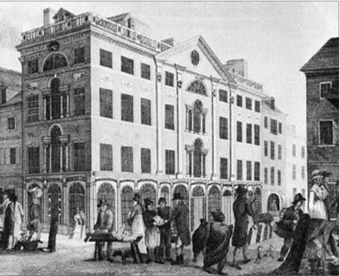
The scene in 1799 at the corner of Third and Market in Philadelphia.
